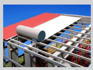
**03.** On placing the next sheet parallel to the first, making the side overlap and staple the edges together.
