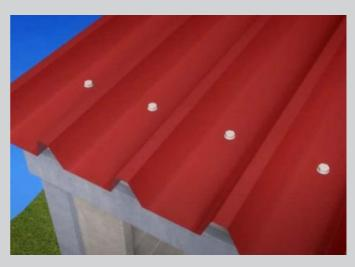
**02.** Place the metal sheet on top of the insulation sheet and fix with metal screws
